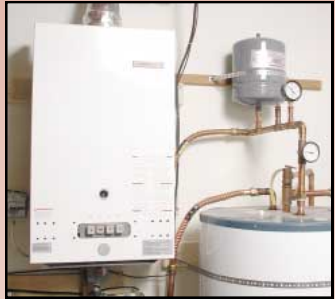
Sometimes the Maine winter is relentless—an AquaStar tankless water heater fills in when the sun doesn't shine.
