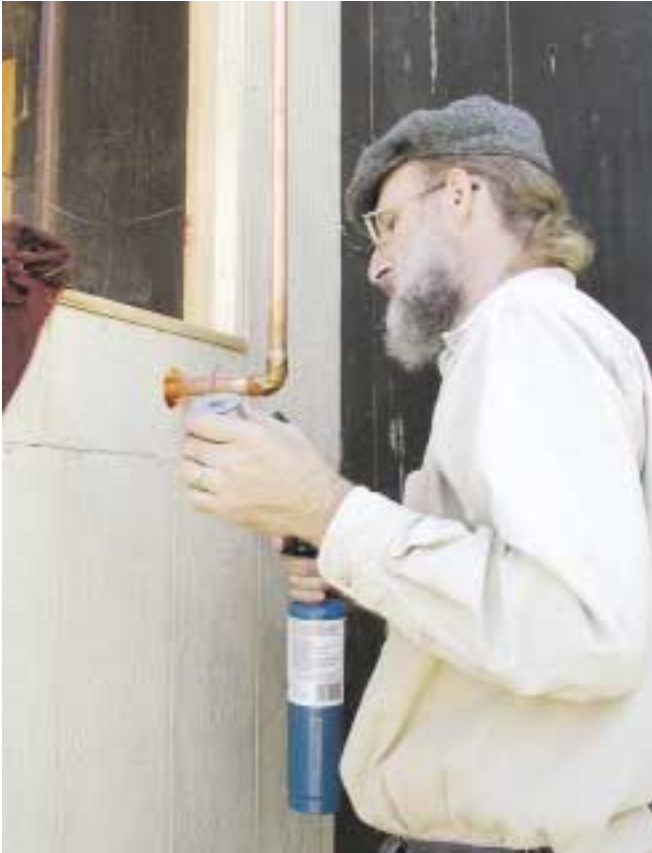
Guy Marsden installed the whole solar hydronic heating system himself.
