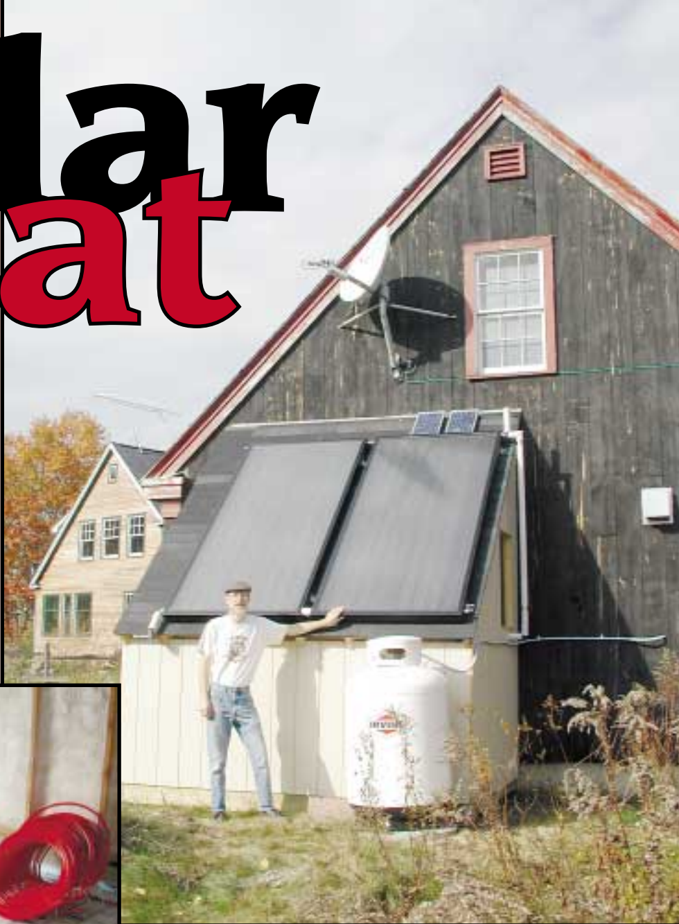
The author with the solar thermal panels that heat his workshop's floor.
